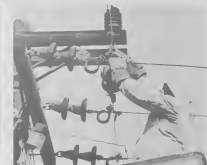
Double gloves (rubber inside leather) are used here by Ramiro Quandt when working on high voltage lines. Ramiro Quandt ta usa handschoen dobbel (di rubber y cuero) pa traha cu linja di alto voltaha.
